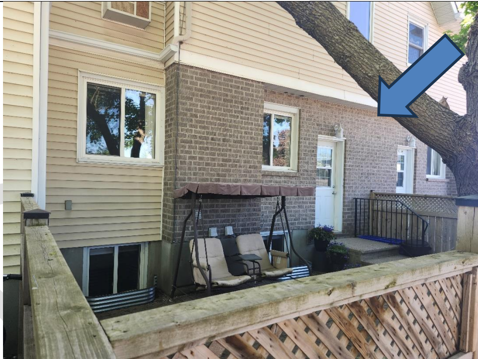
Exterior wall lighting
