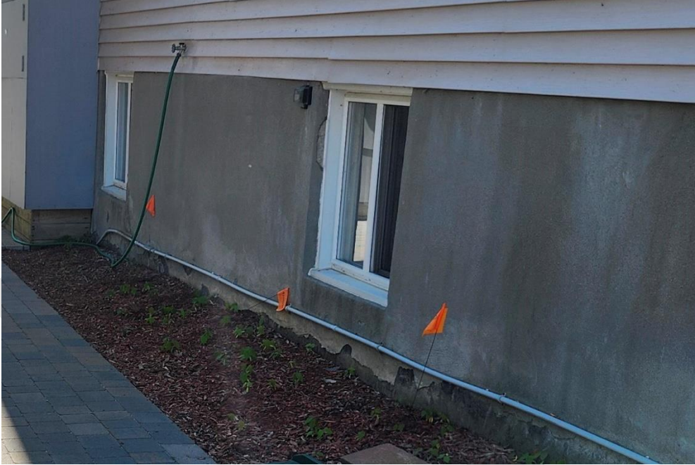
Exposed parged foundation, minor cracking and spalling at time of site
