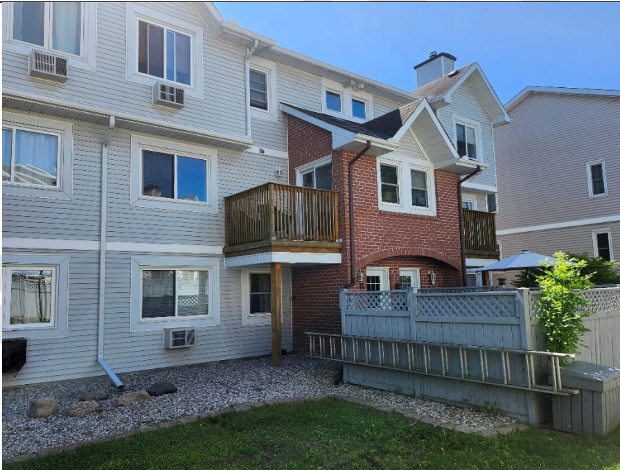
Minimal Brick on 315, on the 2 storey entry elevations.
