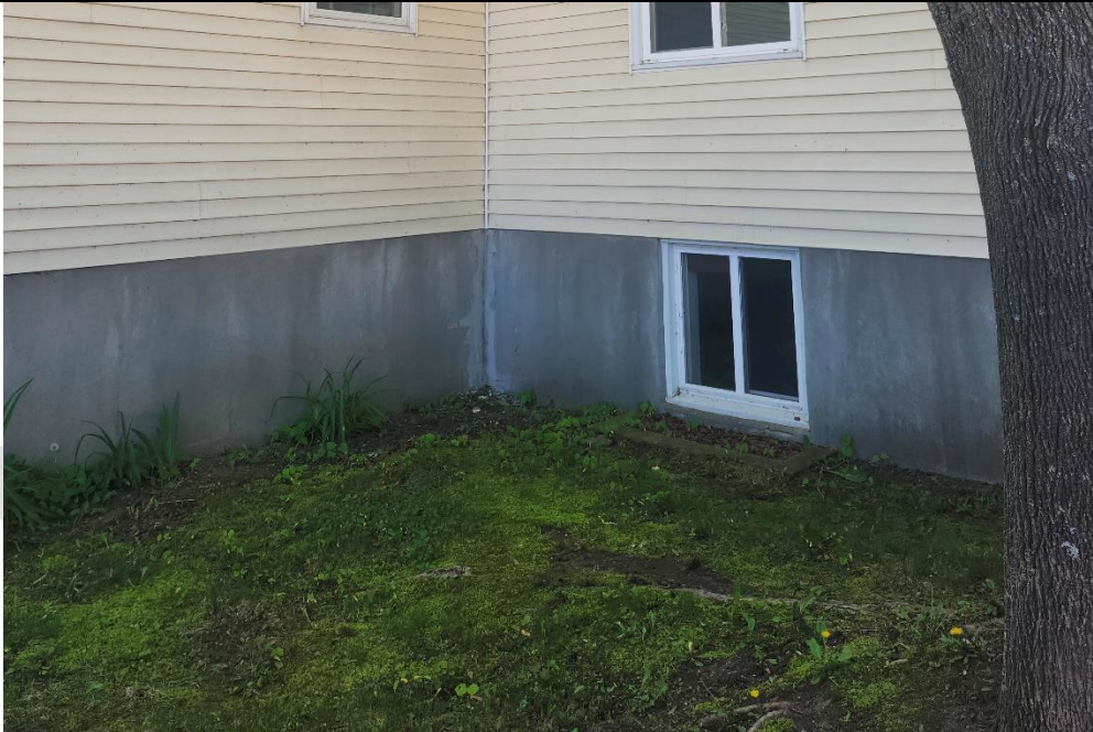
Exposed parged foundation, minor cracking and spalling at time of site
