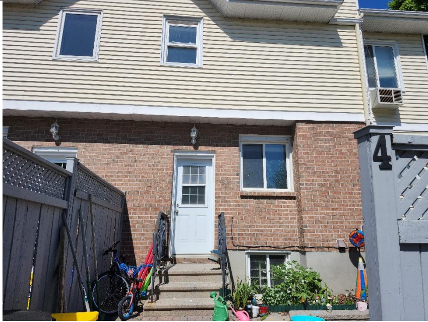
Standard Brick coursing on 1 st floor entry elevations.
