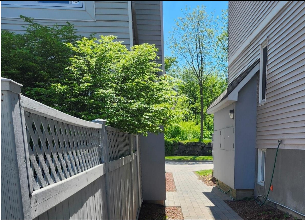
Electrical panel build outs
