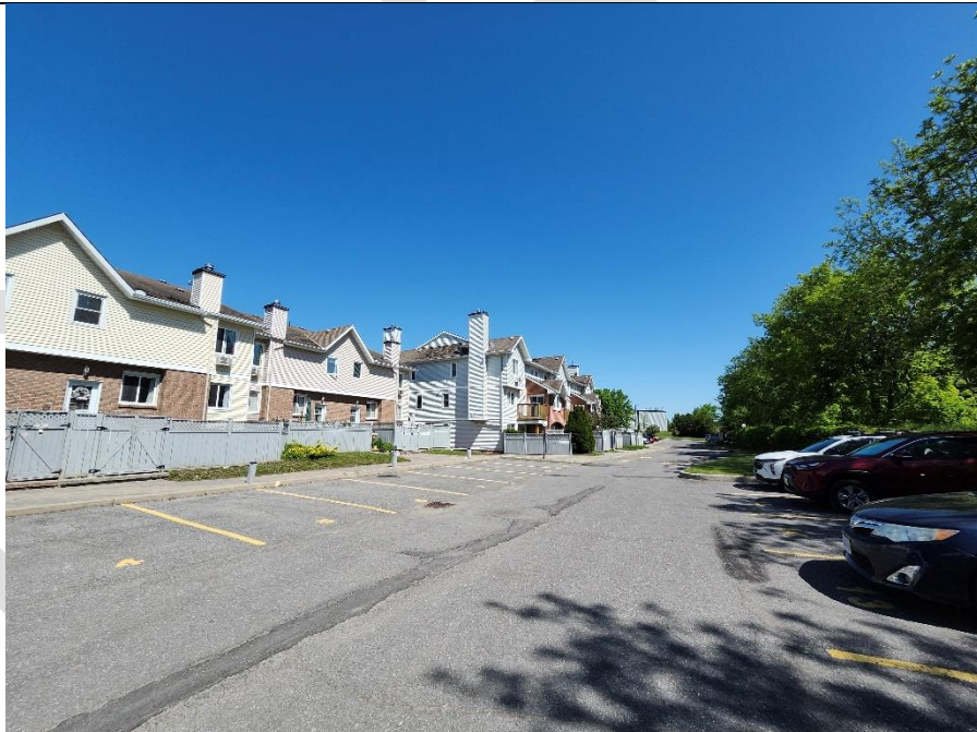
Repair has been completed
