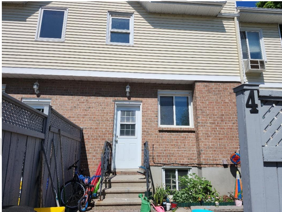
Original concrete with Guards and railing installed.
